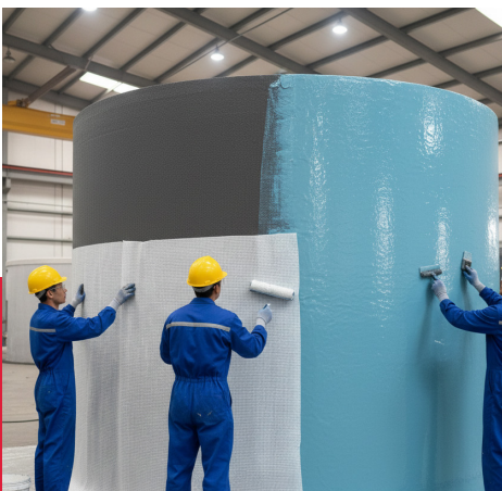
WATER TANK FIBER LAMINATION
