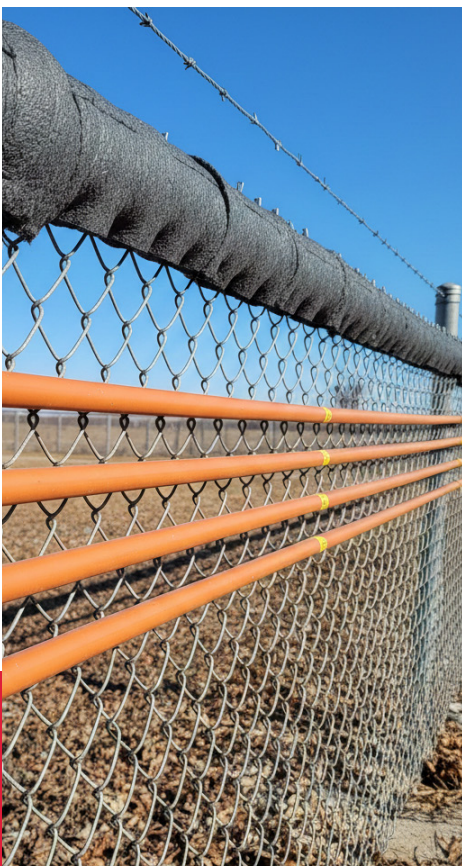
INSULATED CHAIN FENCE
