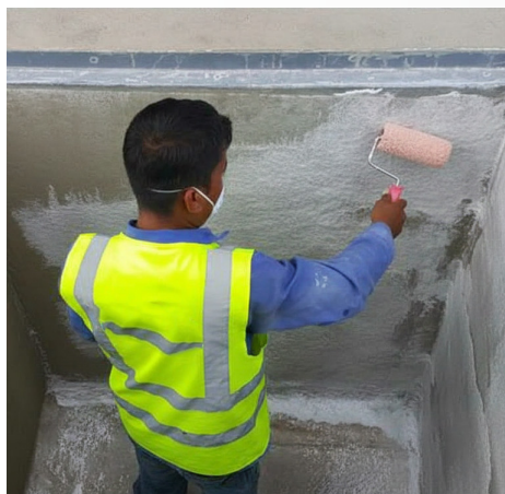
MANHOLE LAMINATION
