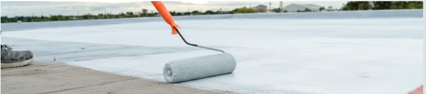
POLYURETHANE WATER PROOFING
