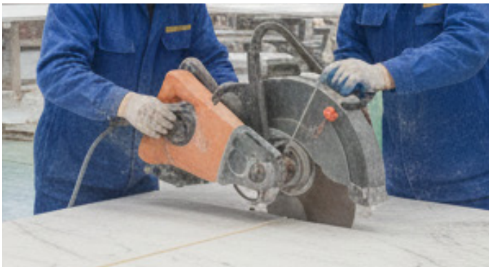
MARBLE AND GRANITE WORKS
