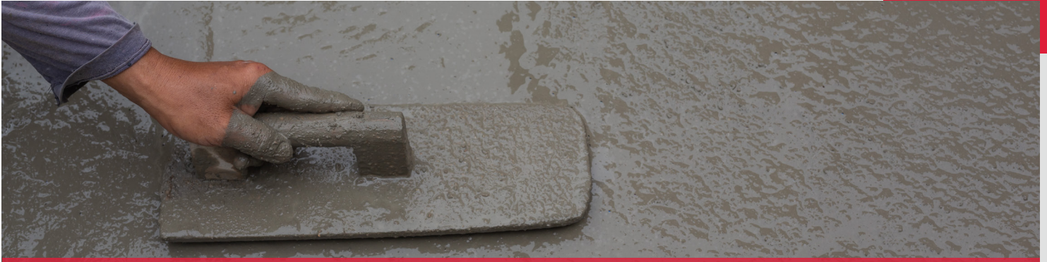
CEMENTITIOUS WATER PROOFING
